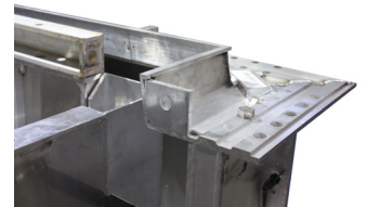
Header Forms placed on Jacket Forms.
