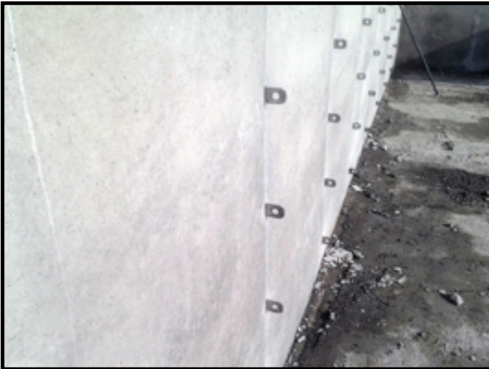
New Forms with the Pour Ready Process
