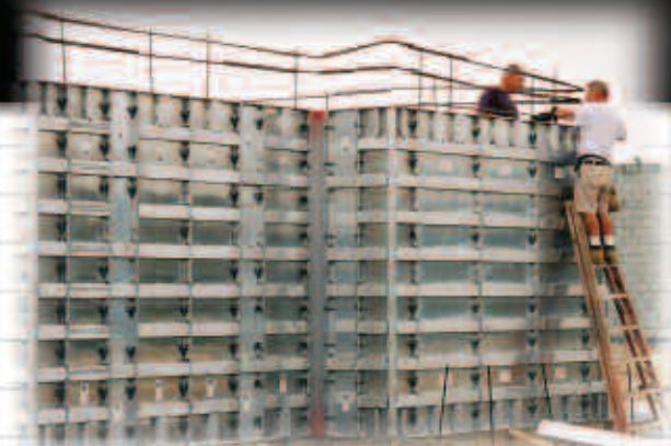
Precise Forms are designed to allow for stacking and are compatible in most form orientations.
