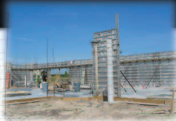
Garage door headers poured monolithically
