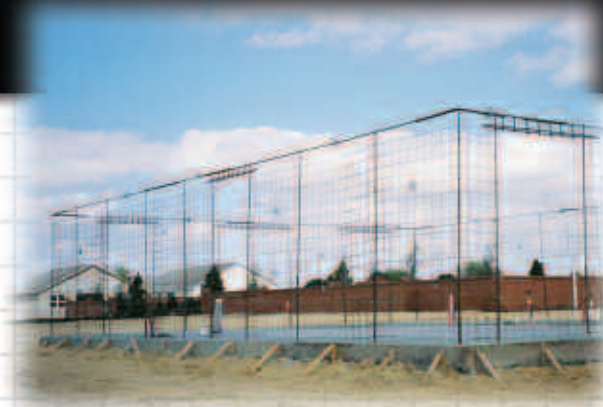
Structural reinforcing placed prior to forms setting
