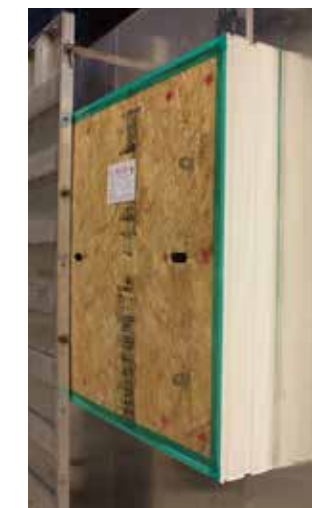
Cast in Place Bucks come with glass sash protected by packing and plywood brace.
