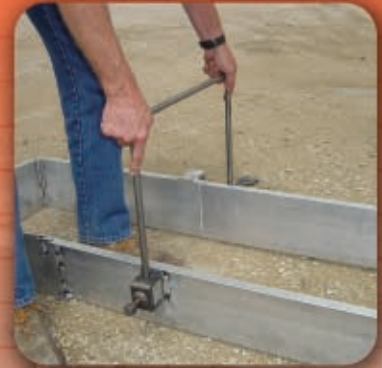
Insertion of the support spacer bar allows depth of footing to be set.
