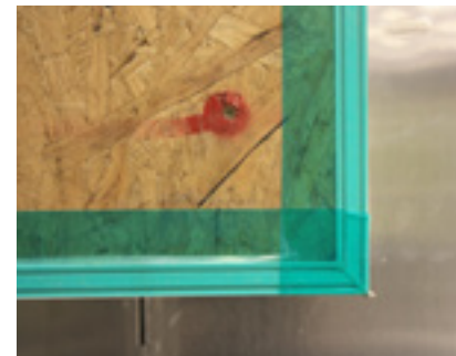
Interior and exterior vinyl unit protected from concrete by tape.
